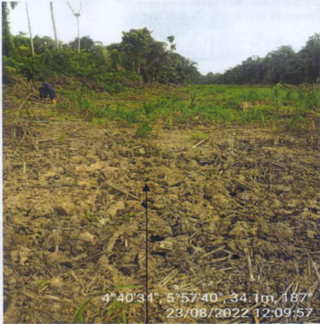
SPILL POINT BEFORE EXCAVATION
